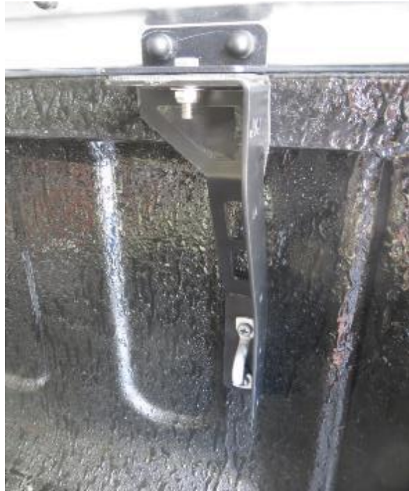
Figure 18: Rear-Right Support Bracket Installed
